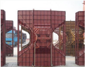
I-beam formwork
