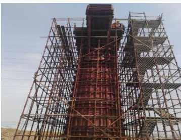
Overpass column formwork
