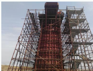
Overpass column formwork
