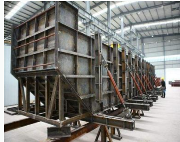
Overpass bent cap formwork
